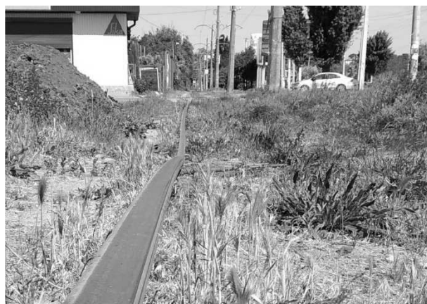
Fig. 3 Actual condition of the geometrical position of a track in terms of buckling occurrence
